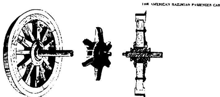
Figure 7.33 A wooden, cast-iron, and wrought-iron 16-inch-diameter wheel used on the New Jersey Railroad and Transportation Company around 1834
