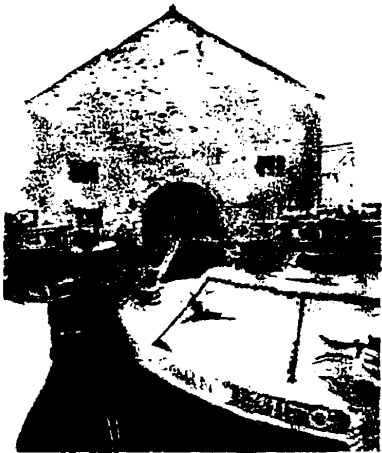
Narrow boats entering building.
